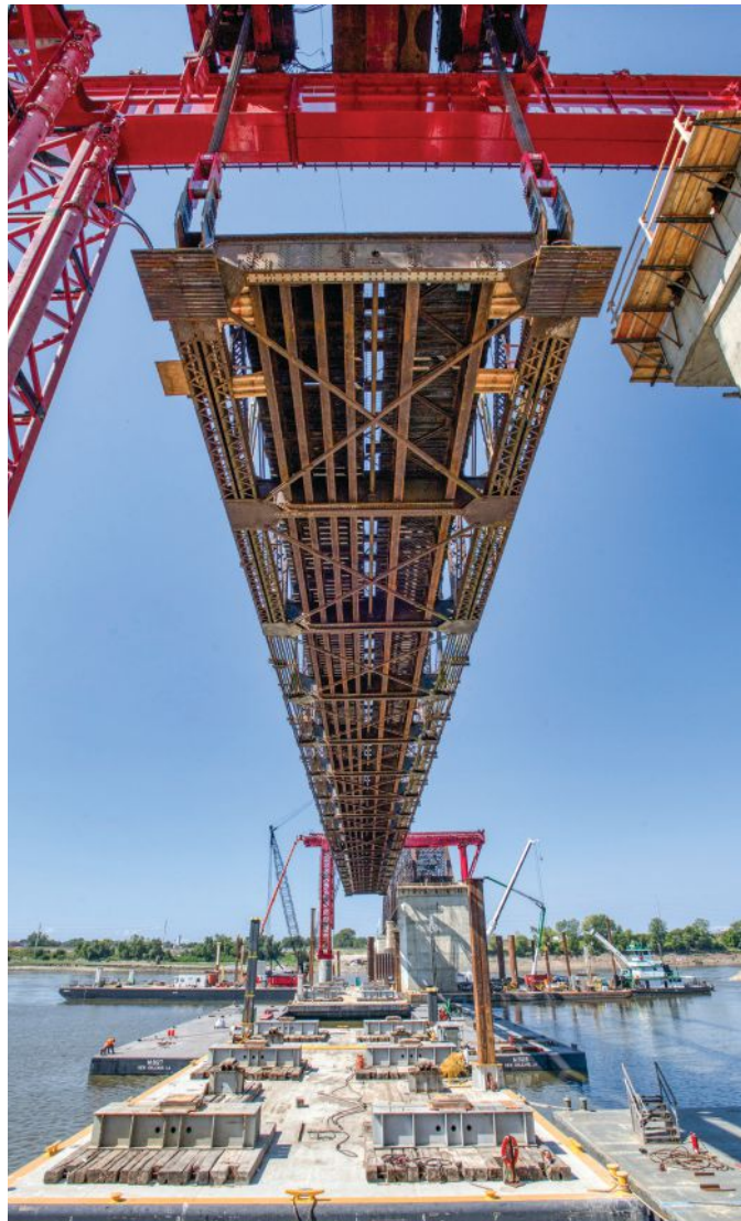
Key aspects of the span change-out included strengthening the existing truss chords for removal, strengthening the existing piers for the gantry system, placing the gantry system for lifting and sliding the spans, and maintaining barge stability and maneuverability in and around obstacles in the river while positioning the truss under the gantry system.
