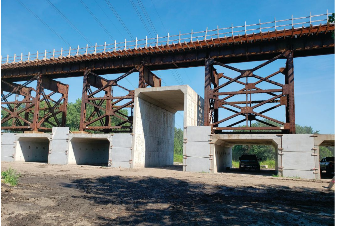
above: Much of the east approach is located within the floodwall limits on the Illinois side of the river. The steel girder trestles spanning 745 ft were originally constructed in 1902, with their condition warranting annual inspection.
