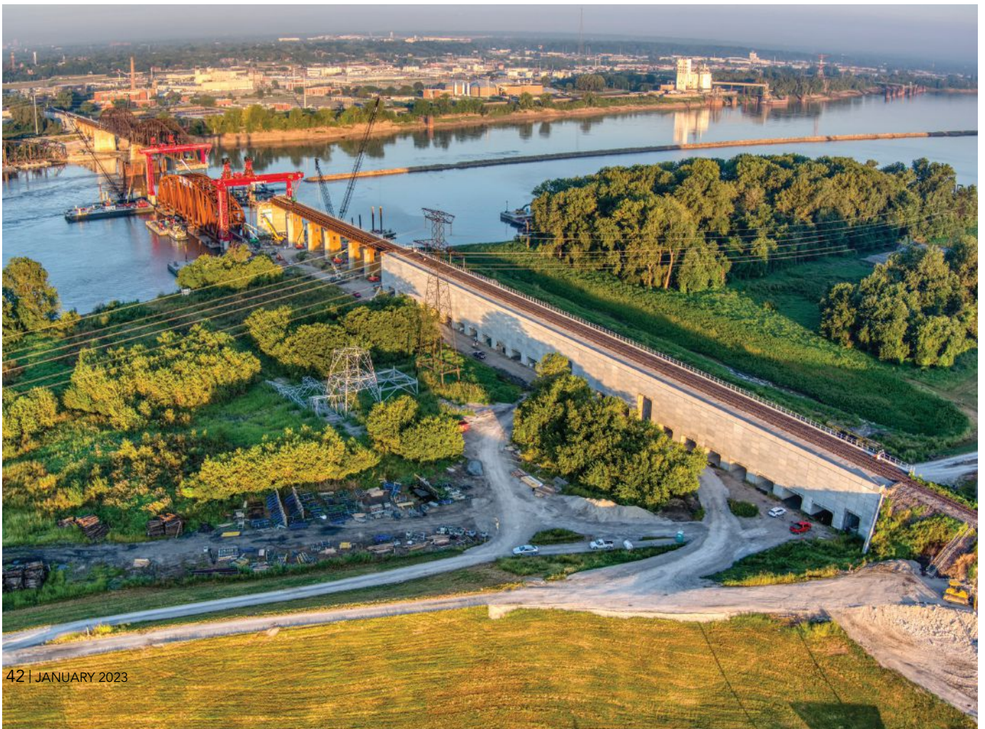
above: Much of the east approach is located within the floodwall limits on the Illinois side of the river. The steel girder trestles spanning 745 ft were originally constructed in 1902, with their condition warranting annual inspection.
