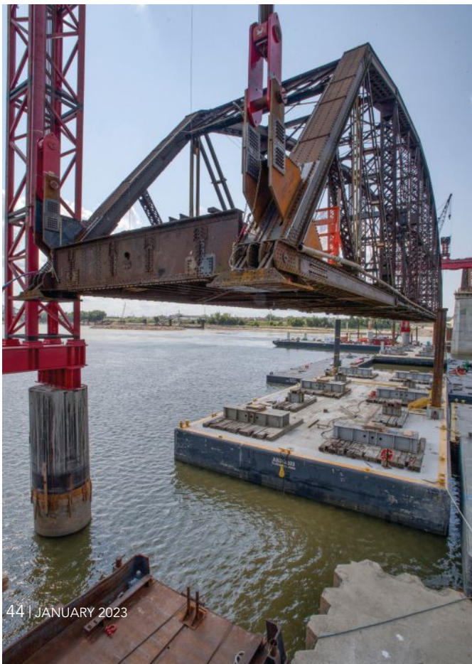
Key aspects of the span change-out included strengthening the existing truss chords for removal, strengthening the existing piers for the gantry system, placing the gantry system for lifting and sliding the spans, and maintaining barge stability and maneuverability in and around obstacles in the river while positioning the truss under the gantry system.
